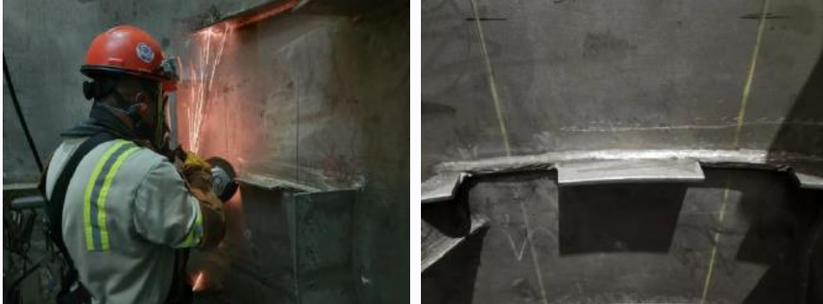
Parts of the original tray supports are cut away because they interfere with the installation of supports for the new liquid and gas distributors between beds #3 and #4
